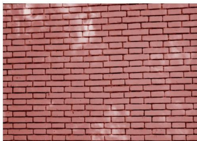
(a) Brick wall
